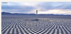
The 110 MW Crescent Dunes Solar Energy Project, Tonopah, Nevada
